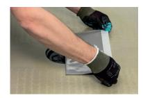
8. You can also seal the floor drain with a self-adherent Kiilto Kaivolaippa reinforcement. Place Kiilto Kaivolaippa on a dry, primed surface and press carefully into position. Cut a hole into it according to the drain manufacturer's instructions and press the tension ring into position.
