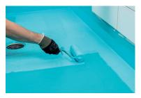
**5.** Roll a second coat of Kerafiber and allow to dry for 6-12 h/colour change before tiling. Check the thickness of the Kerafiber layer. Add Kerafiber on top of thin and/or porous spots and allow to dry properly. The total consumption of Kerafiber should be at least 0.8 l/m² and the layer thickness 0.5 mm.
