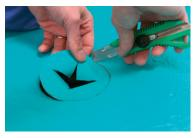
**6.** After the waterproofing membrane has dried, cut a round hole for the floor drain: ensure that the diameter of the hole is at least 40 mm smaller than the diameter of the floor drain, so that the rim of the Kerafiber layer stretches over the seal in the drain (follow the drain manufacturer's instructions). The thickness of the Kerafiber layer around the floor drain should be a minimum of 1.2 mm.
