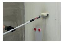
1. Prime dry and dustless walls with Kiilto Keraprimer or Kiilto PrimeOne. Dilute Kiilto Keraprimer with water 1:1. Allow to dry for at least 30–60 minutes before waterproofing.
