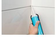
**14.** Wipe away any excess tile grout from the corners, and seal the corners and pipeline inlets with Kiilto Saniteettisilikoni. Wait until the next day before using your new bathroom. If you have an underfloor heating, wait for a week before gradually bringing the system up to its operating temperature.
