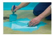
**3b.** Apply waterproofing membrane around the floor drain (approx. 40 x 40 cm area), and turn the prepared floordrain patch over the drain. When using a separate sealing flange, contact our technical support or consult your drain supplier for instructions.
