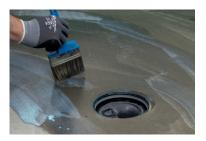
1. Prime dry and dustless floor with Kiilto Keraprimer or Kiilto PrimerOne. Allow to dry for at least 30-60 minutes before waterproofing.
