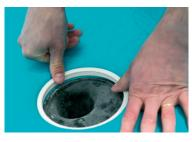
**7.** Press a suitable tension ring into position. Cut off any excess Kerafiber under the ring.
