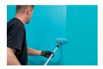
**5.** Roll a second coat of Kerafiber and allow to dry for 6-12 h/colour change before tiling. Check the thickness of the Kerafiber layer. Add Kerafiber on top of thin and/or porous spots and allow to dry properly. The total consumption of Kerafiber should be at least 0.6 l/m² and the layer thickness 0.4 mm.
