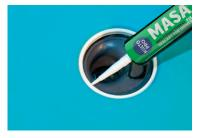
11. Seal the junction between the tension ring and the floor drain with Kiilto Masa Fix and sealant. Kiilto Kaivolaippa has been tested and approved in terms of its compatibility with the most common floor drain types.
