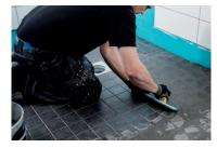
13. Apply Kiilto Lattiasaumalaasti or Kiilto Saumalaasti with a rubber trowel and press it into the joints. Wait for 15-30 minutes and wash away excess grout with a sponge. Use a well-wrung sponge, since too much water may discolour the joints. Wall joints' profile can be finished by using a thick electric
