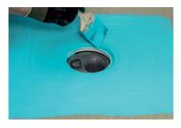
**10.** Apply Kiilto Kerafiber to the entire floor area up to the tension ring.
