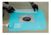
9. Kiilto Kaivolaippa has reinforcements on two sides, apply Kiilto Kerafiber to them. The other two sides must be reinforced with reinforcement tape. Ensure that the tape overlaps with the Kaivolaippa by at least 30 mm.
