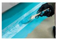
2. Reinforce corners, joints and junctions of different background materials with Kiilto Nurkkavahvikenauha tape. Install the tape onto wet Kerafiber and brush Kerafiber over the tape to ensure wetting. For inside and outside corners, you can use pre-shaped corner reinforcements.
