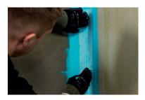
2. Always stir Kiilto Kerafiber before use. Reinforce corners, joints and junctions of different background materials with Kiilto Nurkkavahvikenauha tape. Install the tape onto wet Kerafiber and brush Kerafiber over the tape to ensure wetting.
