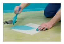
**3a.** The floor drain can be water-proofed with two Kiilto Lattiakaivovahvike floordrain patches. Place one floor drain patch on the floor and brush Kerafiber over it. Place the other patch over the first patch crosswise and brush Kerafiber over it.
